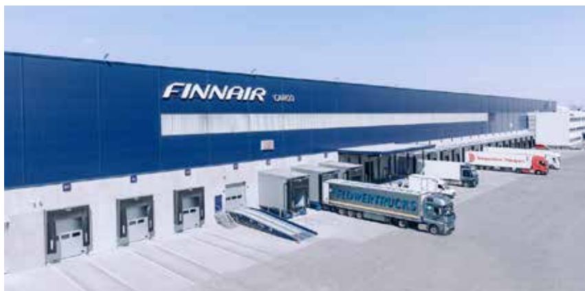
Finnair Cargo's cutting-edge Cool terminal at Helsinki-Vantaa Airport. Photo: Finnair
